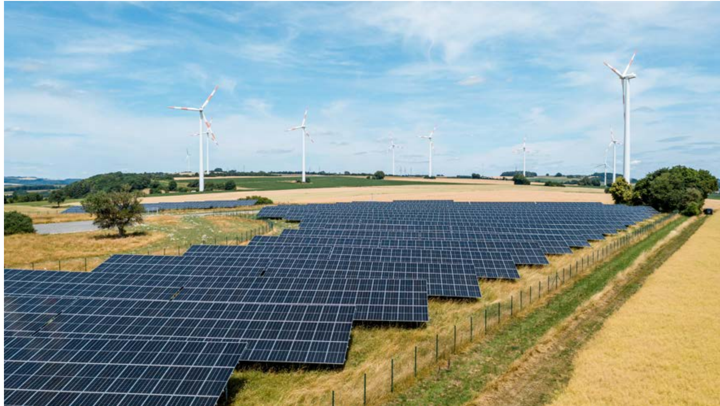
Trianel realises 80 MWp ground-mounted PV systems in the Eifel region
